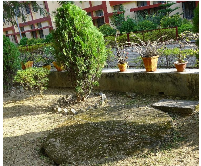
Rain Water Harvesting Pipelines & recharge Pits
