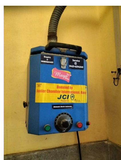
Sanitary pad incinerator
