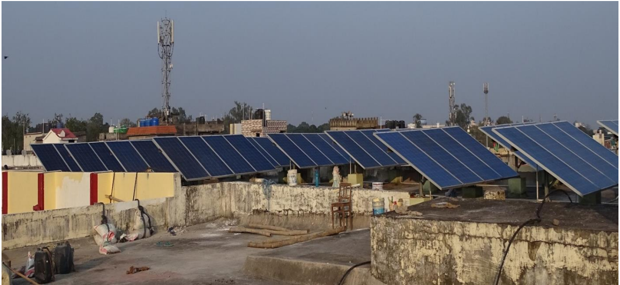
Fig 6 - Solar Panel installed at administrative block, Nirmala College, Ranchi ( Pic. Courtesy: Mr. R.P. Singh, Lead Auditor )
