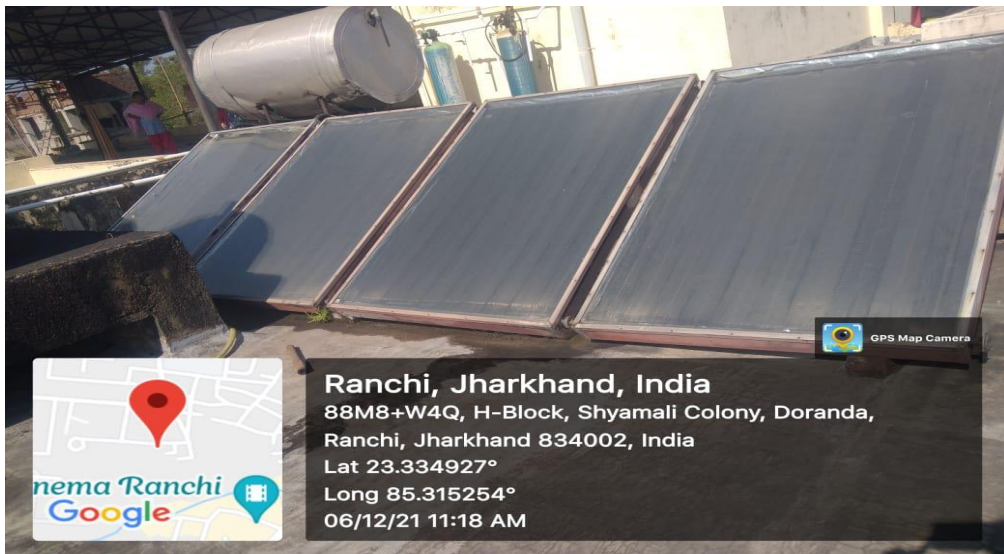
Fig 7 - Solar Heater installed at Staff quarters, Nirmala College
